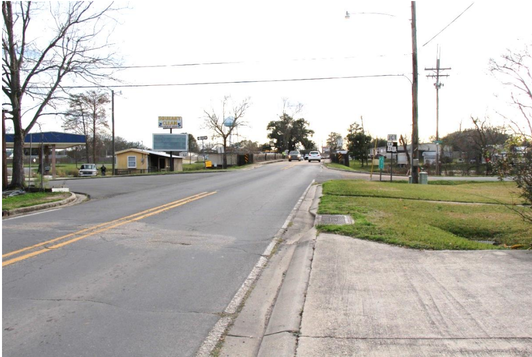
Condition Photo 12: Looking south from the approach span.
