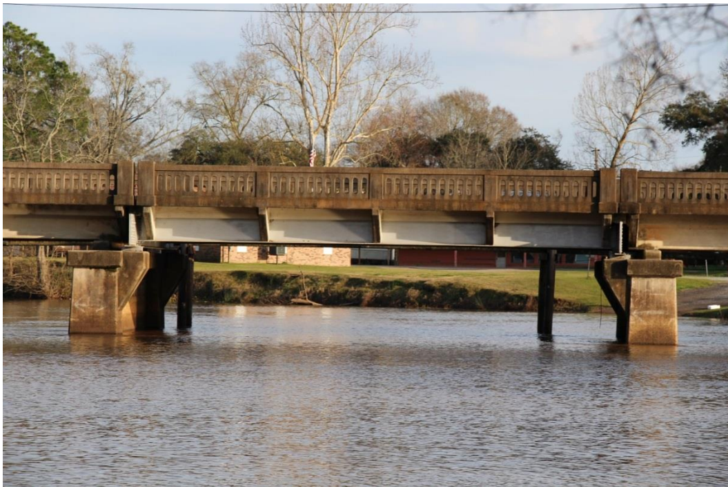
Condition Photo 9: Steel beam removable span.
