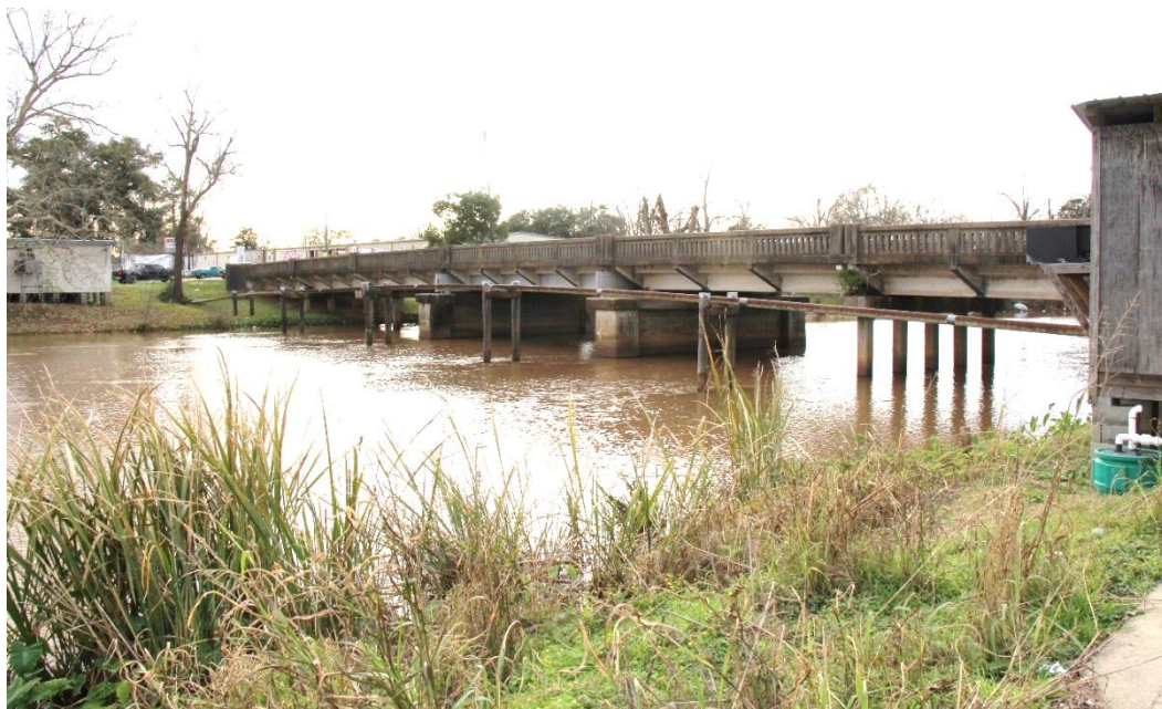
Condition Photo 1: Overview of bridge, facing southwest.
