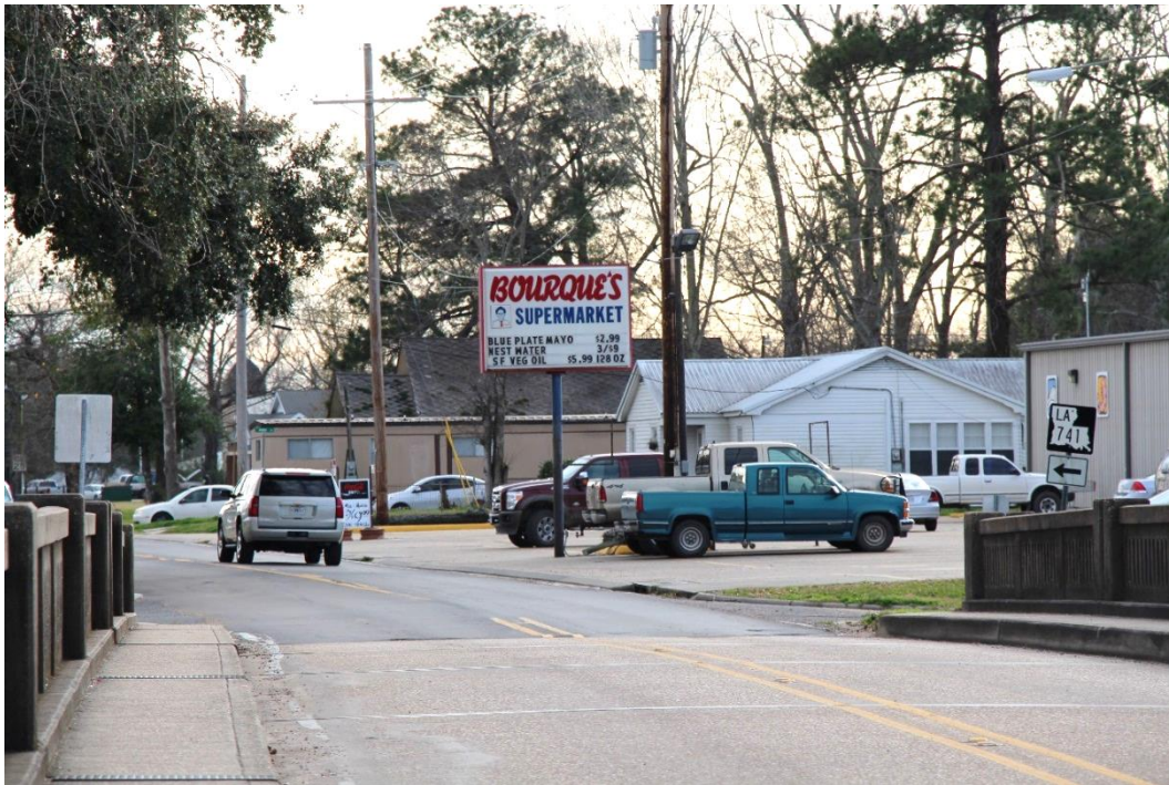
Condition Photo 11: Looking south from the south approach span.
