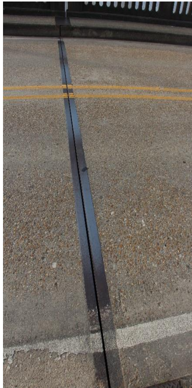
Condition Photo 13: Pier 2, open deck joint in good condition.
