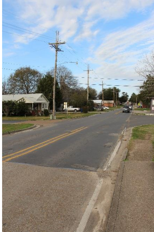
Condition Photo 10: Looking north from the north approach span.
