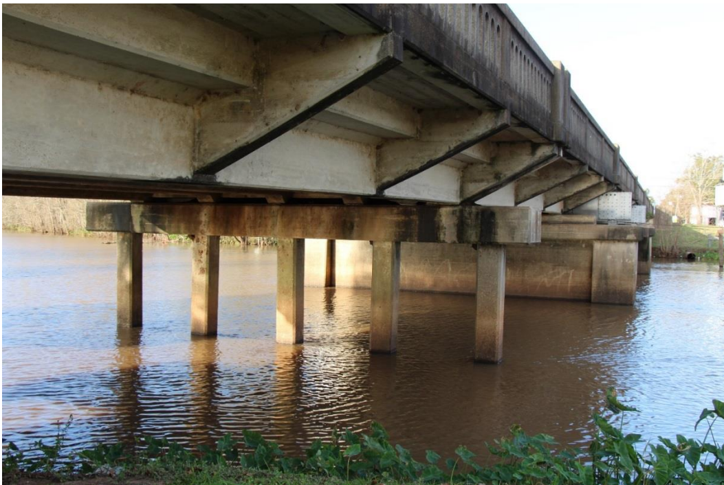
Historic Fabric Photo 1: Concrete substructure, which includes the bents and piers.
